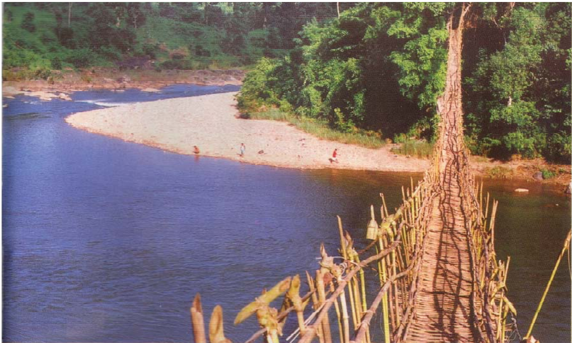
CANE SUSPENSION BRIDGE OVER SIMSANG RIVER
