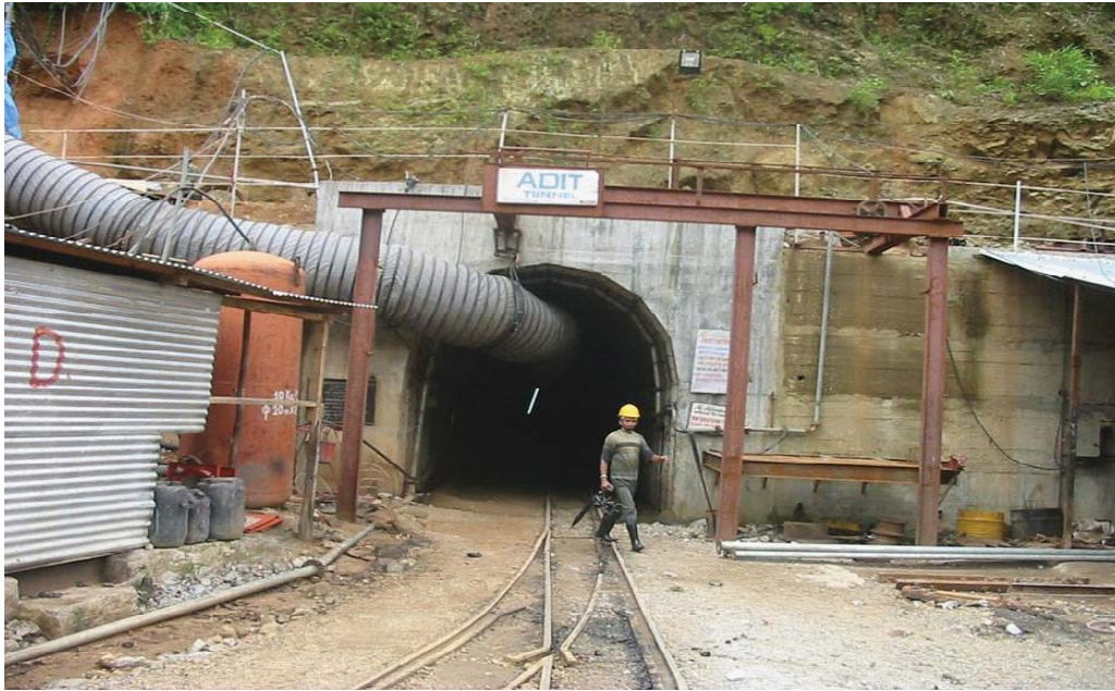
TUNNEL WORK UNDER CONSTRUCTION
